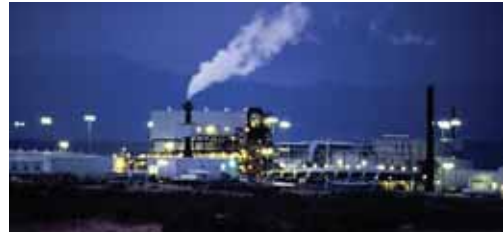
Deseret Chemical Depot
